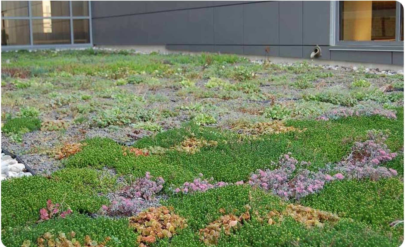
Among other benefits, green roofs reduce the urban heat island effect and increase urban greening.
