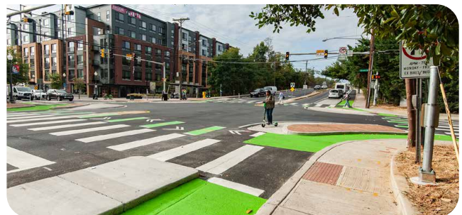
First Mid-Atlantic Region protected intersection, located at Spring Street and Second Avenue
