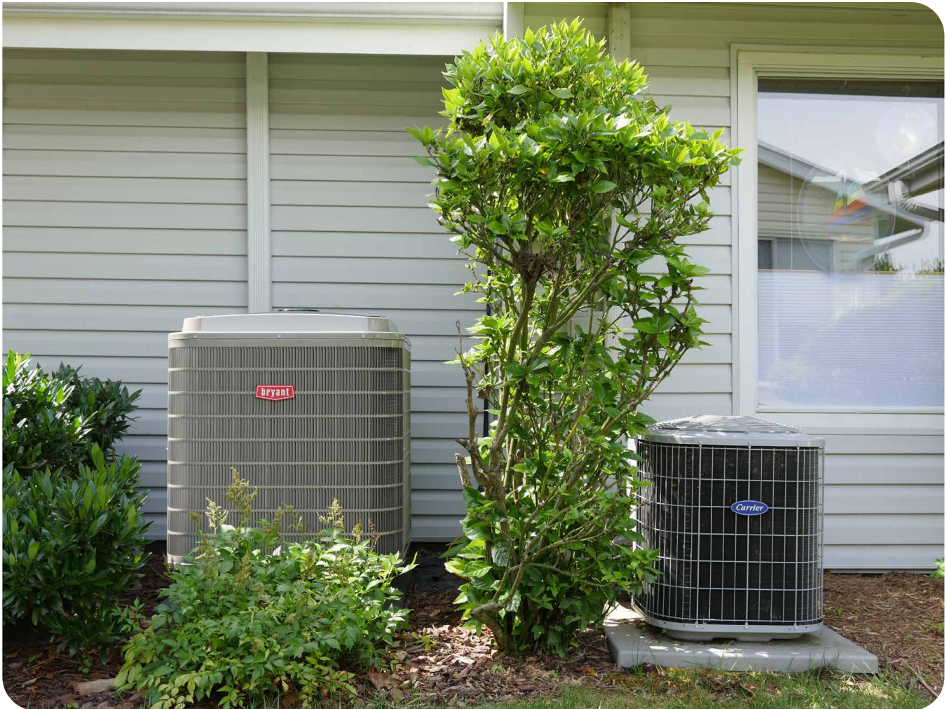
An external unit for a residential heat pump (left), next to a traditional HVAC unit (right).
