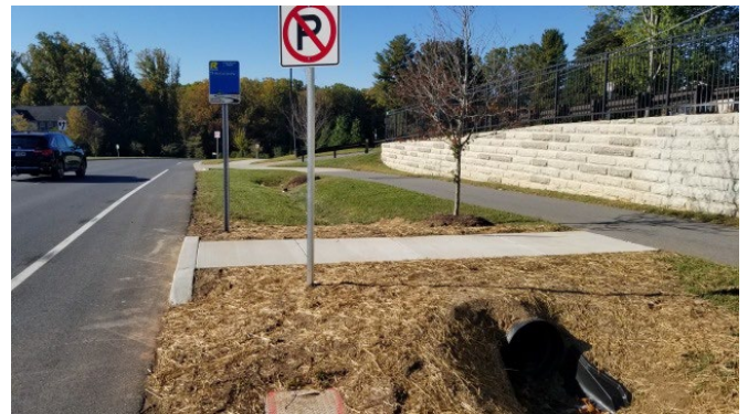
Figure 20 - After conditions with new connection between bus stop and shared use path at Stringtown Road and Gate Rail Road.
