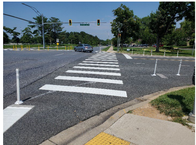
Figure 10 - Montgomery County installed flexposts along Lost Knife Road to slow down vehicle turning speeds in spring 2023. Long term work will be associated with redevelopment of mall property.
