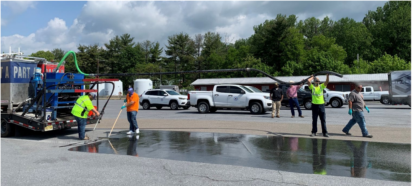
Figure 13 - Contractors demonstrate application process for high friction surface treatment at SHA service yard.
