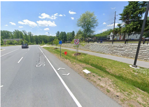
Figure 19 - Before conditions at bus stop at Stringtown Road and Gate Rail Road.
