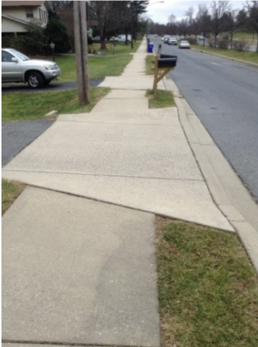
Figure 21 – Example of Non-Compliant Driveway Apron
