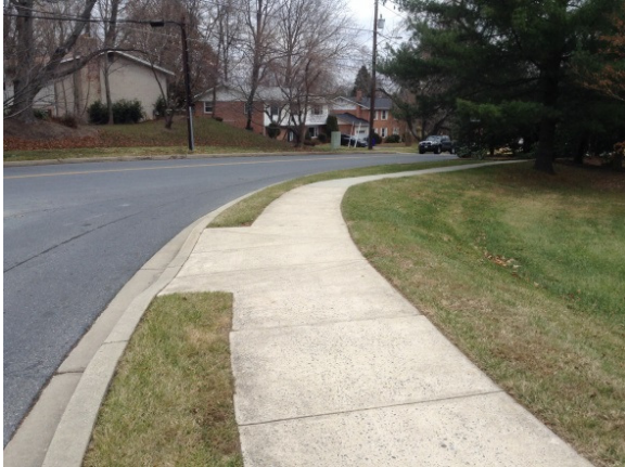
Figure 18 – Example of Non-Compliant Curb Ramp
