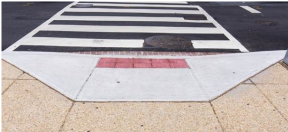
Figure 19 – ADA-Compliant Perpendicular Curb Ramp
