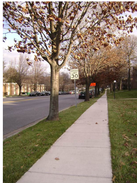
Figure 1 – Example of ADA-Compliant Sidewalk, 4-ft min. width
