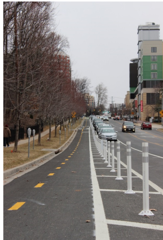
Figure 17 – Example of Two-way; Protected Cycle Track along Woodglan Drive, Montgomery County
