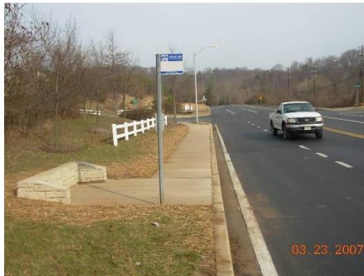
Extensive sidewalk, ramp and knee wall.
