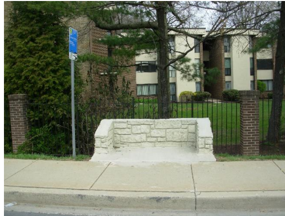
Landing pad and knee wall (double as a bench and barrier for wheelchairs).
