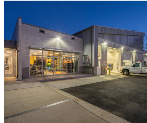
(above and below) Washington Gas - Fleet Facility Addition LEED Gold | Photo: Nomoi Design LLC.
