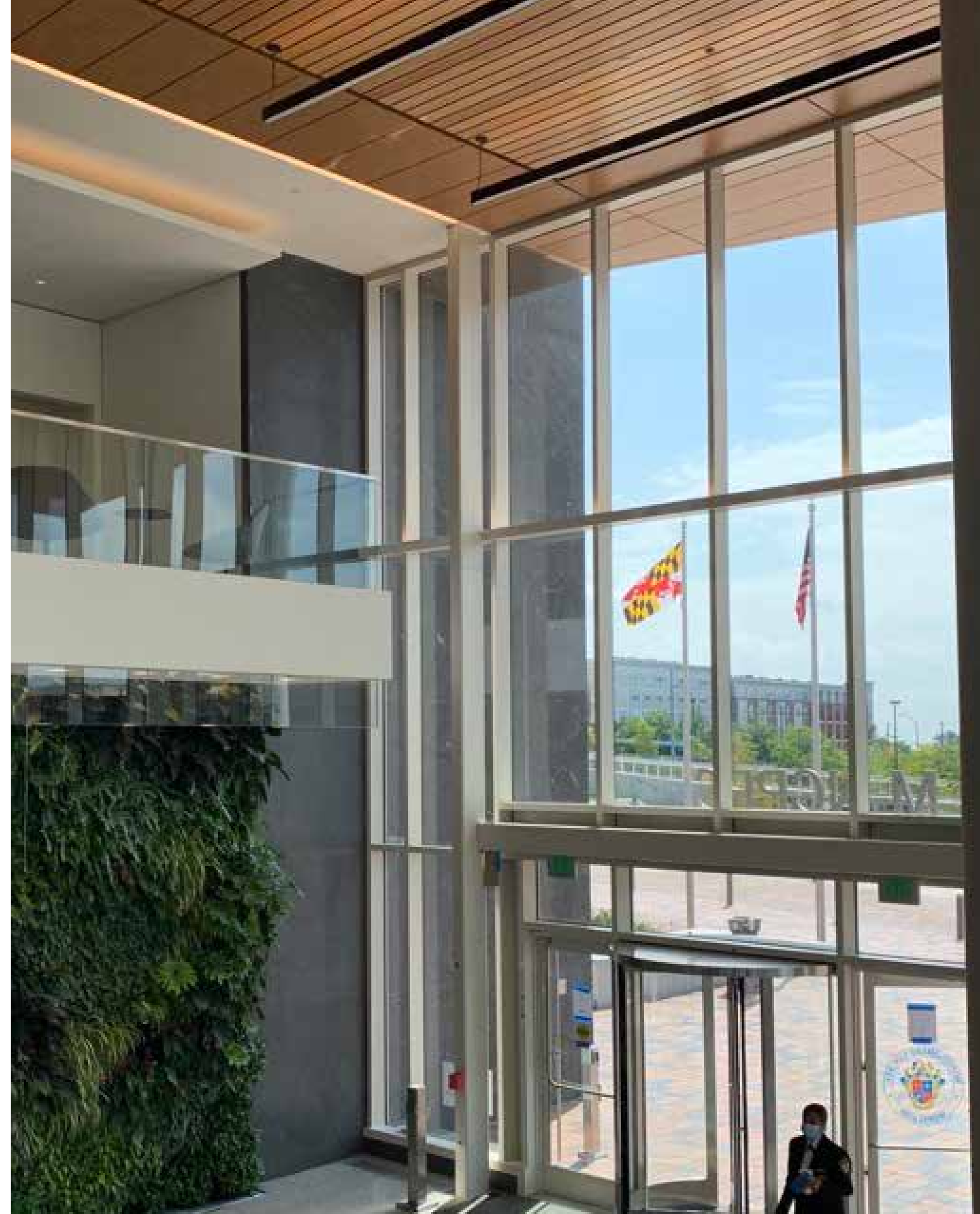
Wheaton revitalization project will achieve LEED platinum certification and include an efficient mechanical system, solar panels, EV charging station sites, and more
