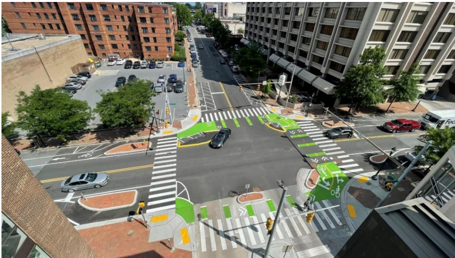
The County's 3 rd protected intersection installed this year at Cameron and Fenton Streets.
