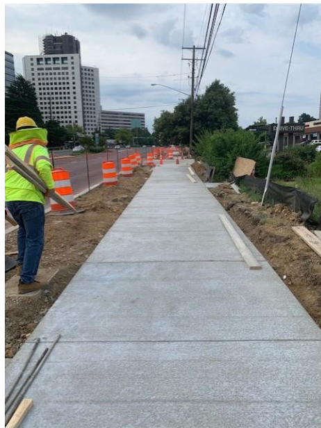
Construction crews installing new sidewalk with additional buffer along Rockville Pike.
