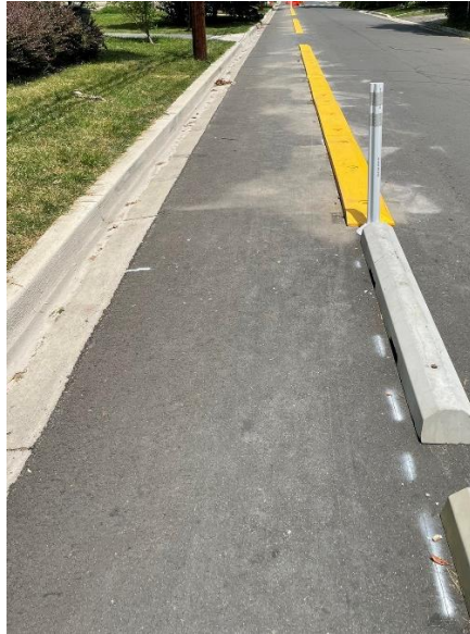
Installation of walking lane along Grove Street
