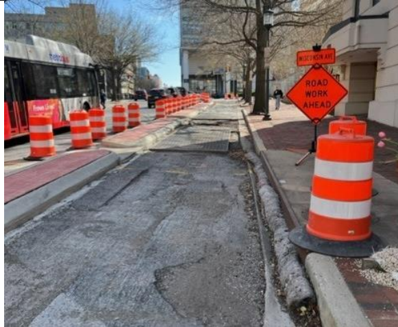
Construction of Montgomery Lane two-way bikeway underway.
