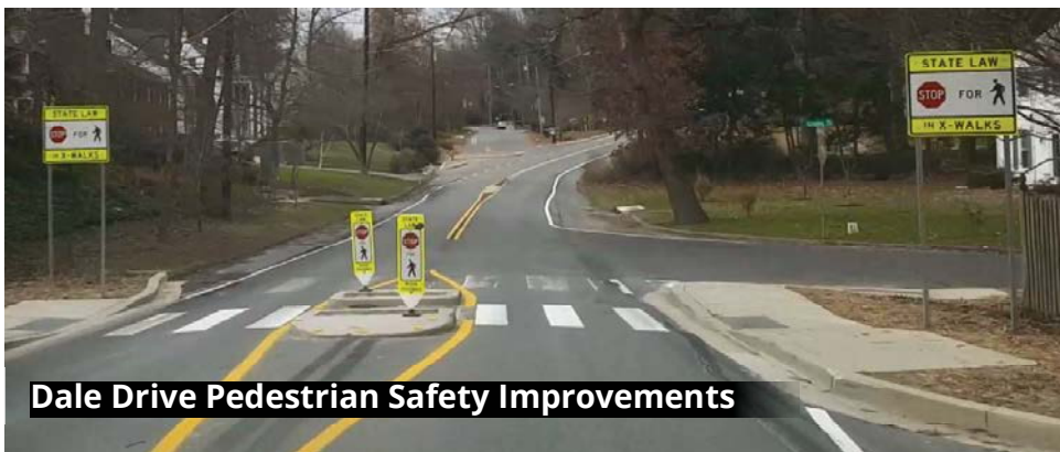
School Crosswalk and Flexposts
