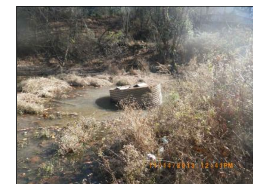
FIGURE 1. REPLACE EXISTING RISER WITH WATERTIGHT CONCRETE RISER.
