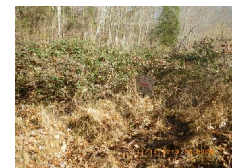
FIGURE 5. CLEAR EXISTING BRUSH AND WOODY VEGETATION FROM DOWNSTREAM EMBANKMENT.
