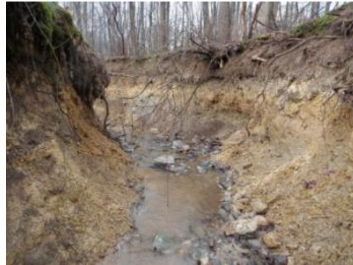
Severely Eroded Bank with Vegetation Loss
