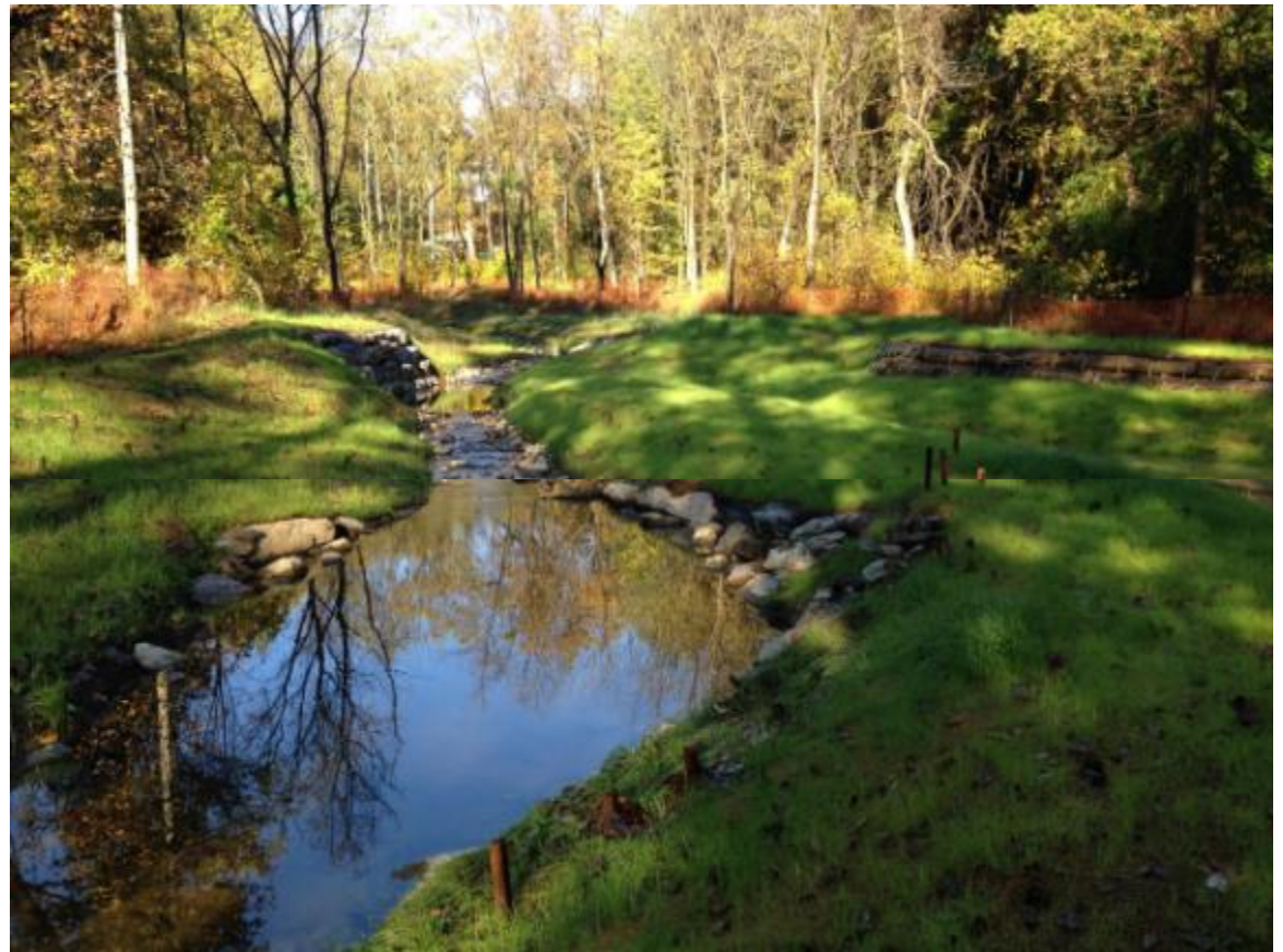
Channel Realignment: Glenora Tributary. City of Rockville. Construction 2014
