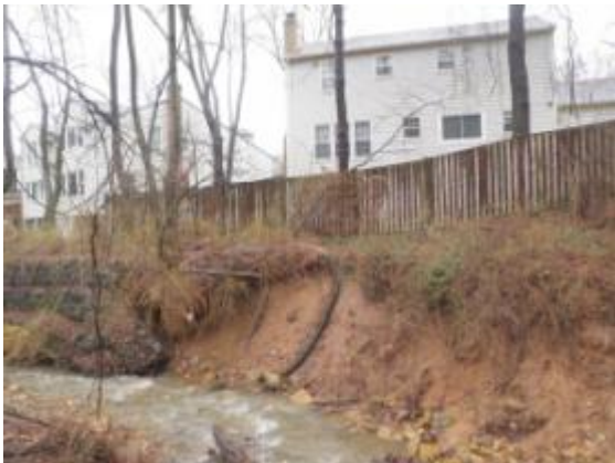
Glenora Tributary: Previous Condition
