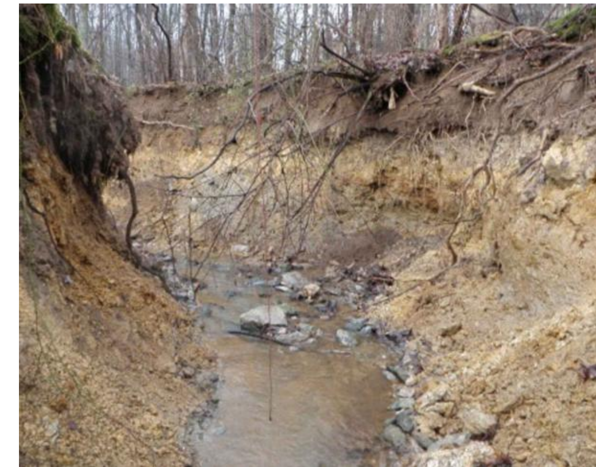
SEVERELY ERODED, DEEP CHANNEL WITH BANKS >6' TALL
