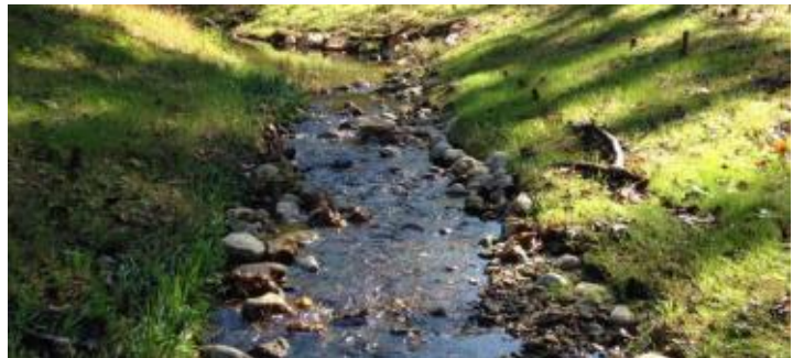
Example of Riffle Grade Control
