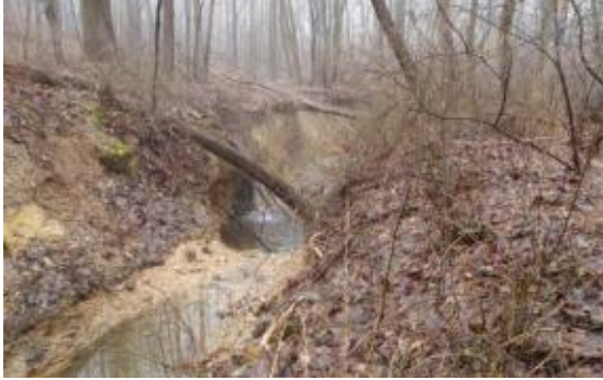
Severe Head Cut Moving Up-stream
