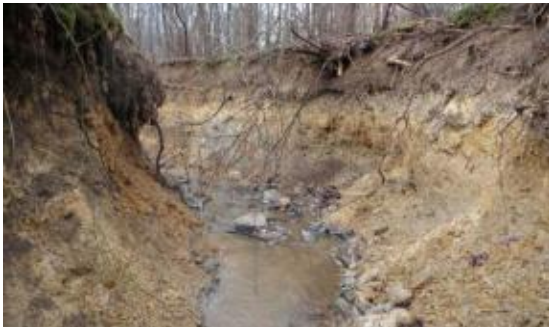
Bank Erosion Ranging From 6-8 Feet
