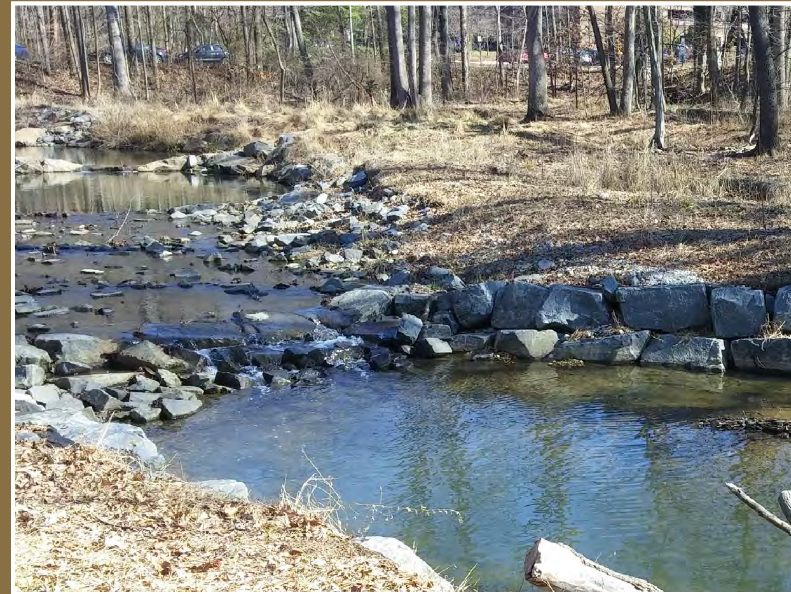
CROSS VANE W/ RIFFLE GRADE CONTROL (CV/RGC)
