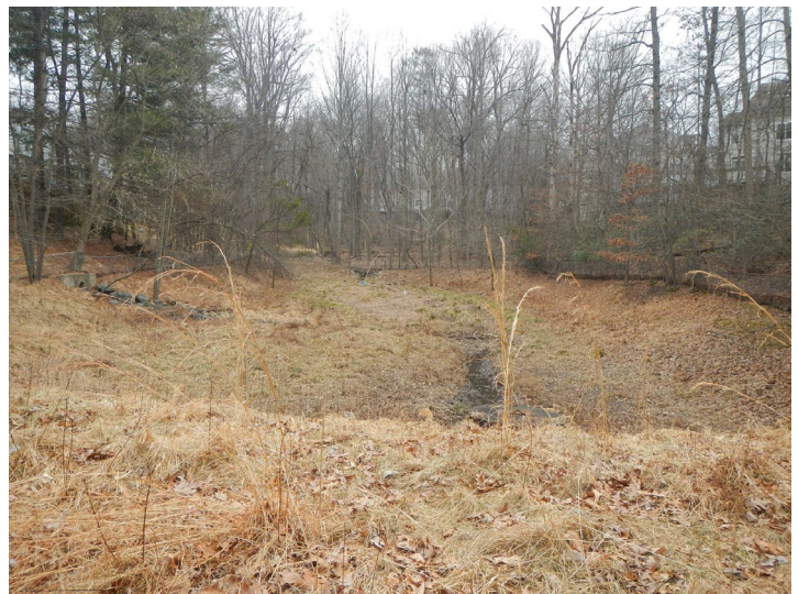
[Photo 3] Overall view of pond facility.
