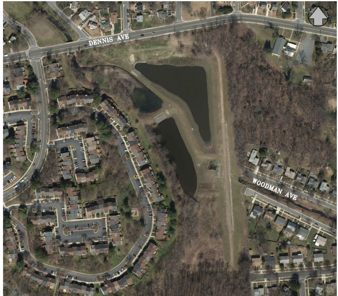
Wheaton Branch Stormwater Pond
