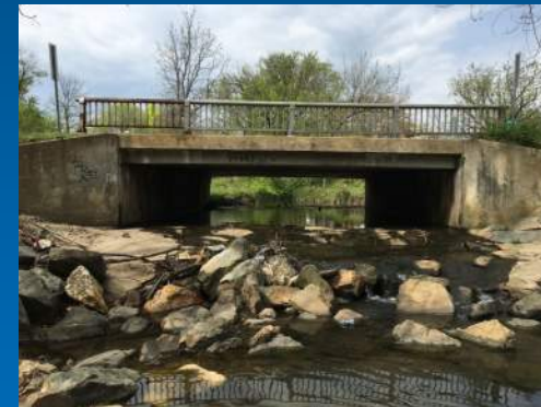
South elevation (looking upstream)
