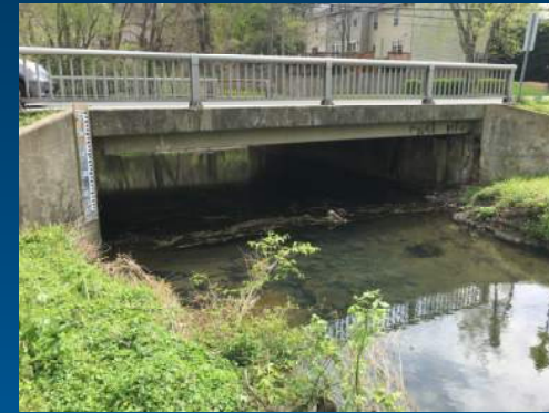
North elevation (looking downstream)
