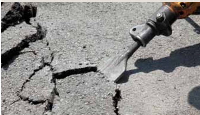
Breaking up pavement
