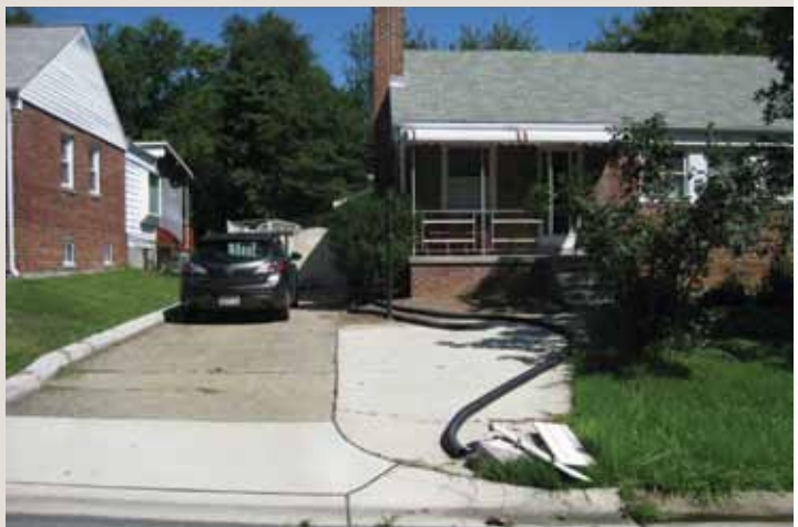
Remove excess driveway and create area to soak in downspout drainage
