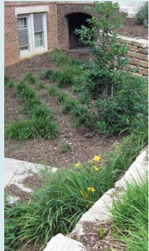
Sidewalk pavement removal - recycled sidewalk into a stacked wall
