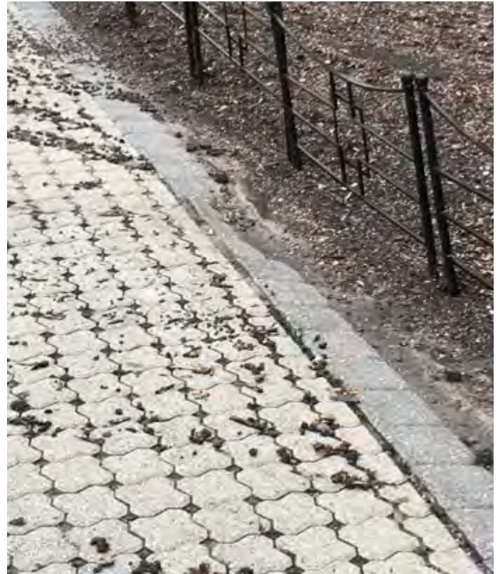
Failing edge restraint caused by improper product and installation using a plastic edging (Refer to aluminum edge restraint detail)
