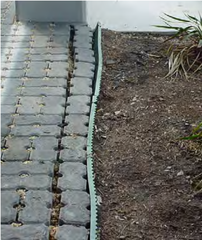
Failing edge restraint caused by improper product and installation using a plastic edging (Refer to aluminum edge restraint detail)
