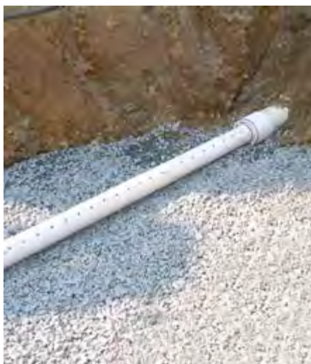
Underdrain pipe is placed on an optional gravel sump.
