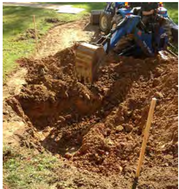
Excavation with toothed bucket
