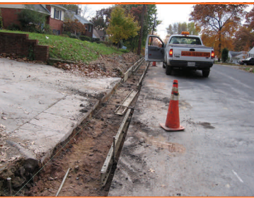
Curb forms being made ready for concrete
