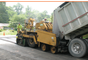
Typical asphalt paving operation
