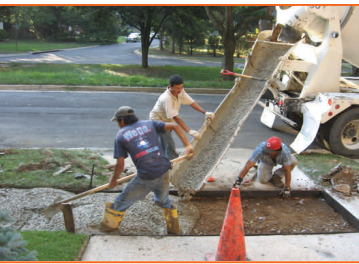
Pouring new concrete into forms
