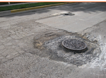
Utilities will be raised to meet new HMA
