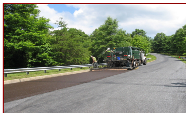
Micro surfacing application
