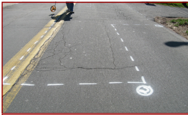
Typical paint markings
