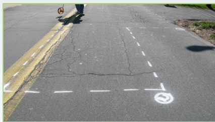
Typical survey paint markings
