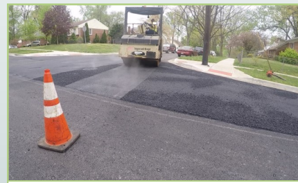
Rollers compact and smooth the asphalt
