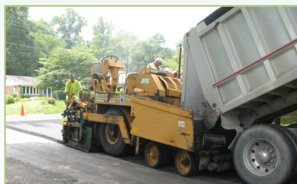
Typical asphalt paving operation
