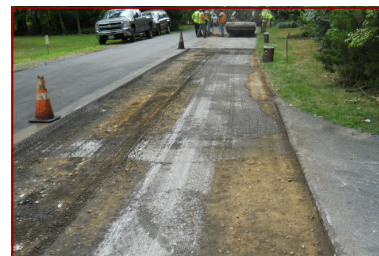
Pavement will be replaced in 2 phases
