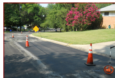
New patch is flush with existing pavement
