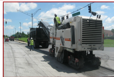
Milling machine excavating
