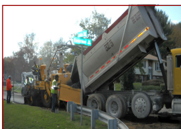
Typical asphalt paving operation.
