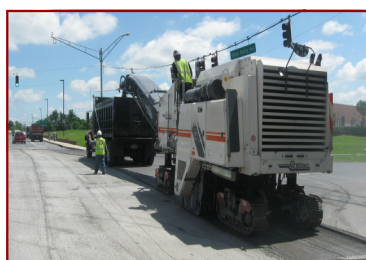
Typical milling operation.
