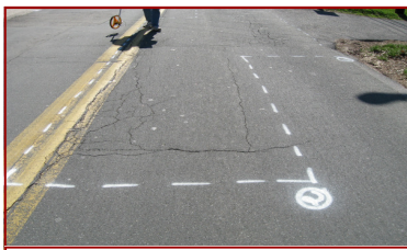
Typical patching paint markings
