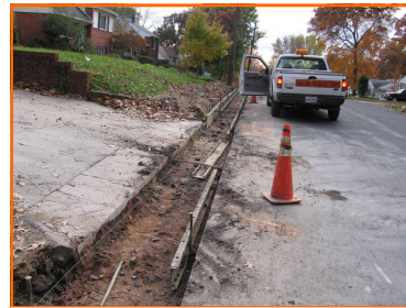
Curb forms ready for concrete
