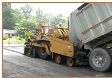
Typical asphalt paving operation
