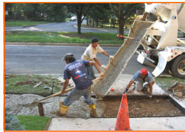
Pouring new concrete into forms
