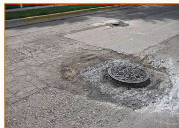
Utilities will be raised to meet new HMA
