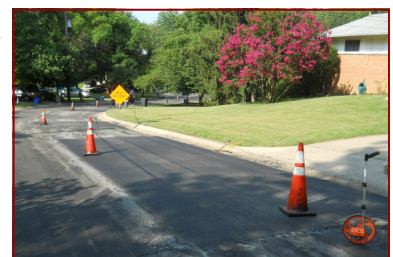
New patch is flush with existing pavement
