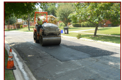
New asphalt is placed and compacted
