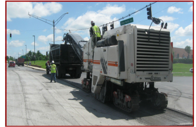
Typical milling excavation operation
