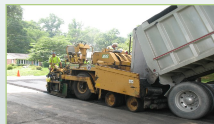
Typical hot mix asphalt paving operation
