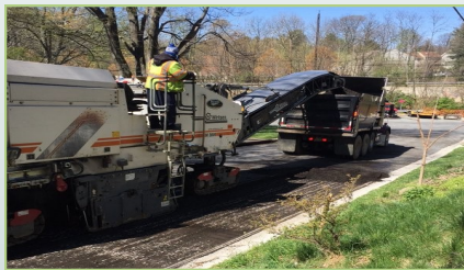
Milling machine patch excavating
