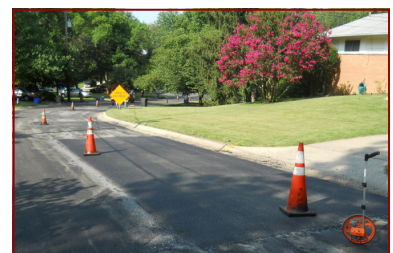
New patch is flush with existing pavement
