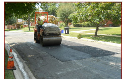
New asphalt is placed and compacted
