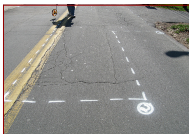
Typical paint markings.
