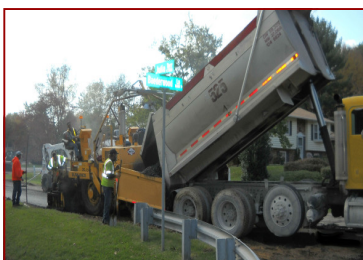
Typical asphalt paving operation
