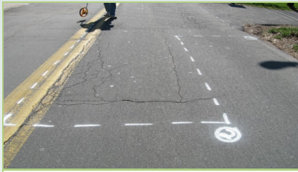
Typical survey paint markings
