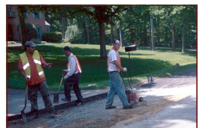
New asphalt is placed and compacted
