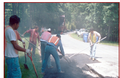
Compacting the sub-grade
