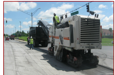
Typical milling operation
