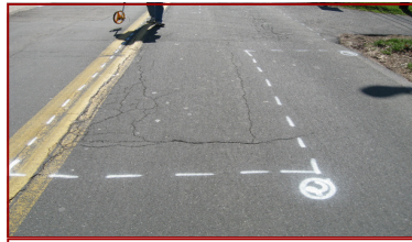
Typical paint markings
