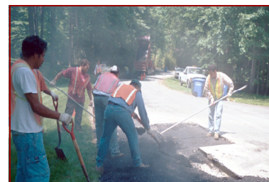
Compacting the sub-grade
