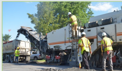
Typical milling operation
