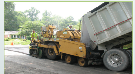
Typical hot mix asphalt paving operation
