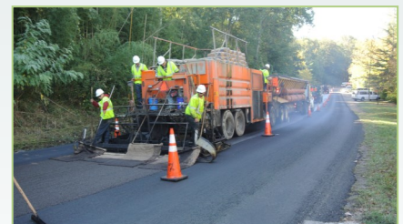
Typical micro-surfacing operation
