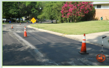
Patching may be necessary prior to resurfacing
