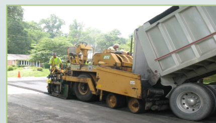
Typical hot mix asphalt paving operation
