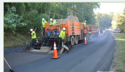
Typical micro-surfacing operation
