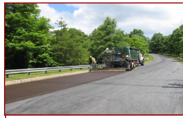
Micro surfacing application
