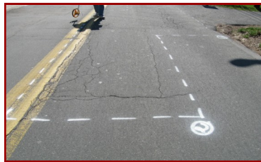
Typical patching paint markings
