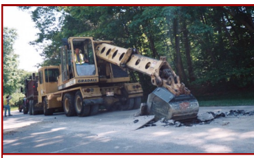
Typical asphalt excavation operation
