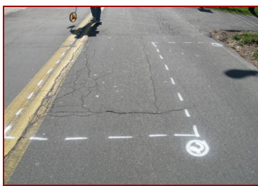
Typical paint markings.
