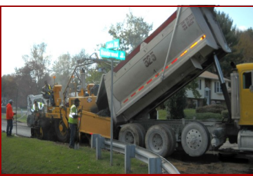
Typical asphalt paving operation
