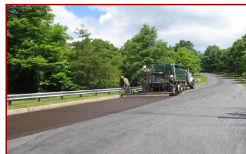
Micro surfacing application
