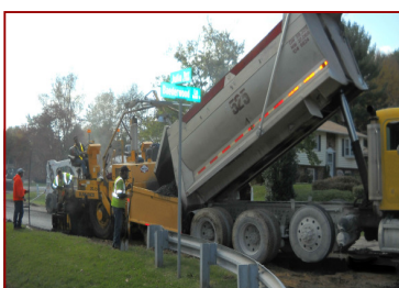
Typical asphalt paving operation
