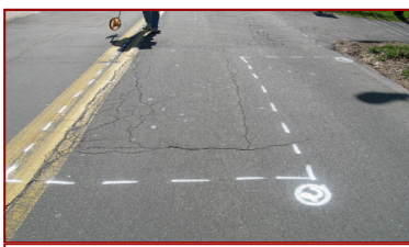
Typical paint markings
