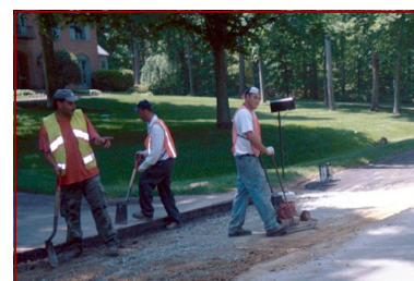
New asphalt is placed and compacted
