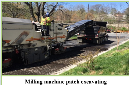
Milling machine patch excavating
