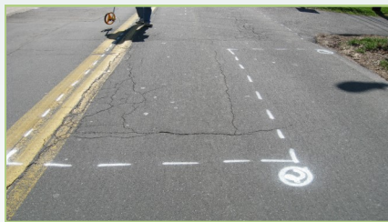
Typical survey paint markings
