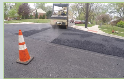
New asphalt is placed and compacted
