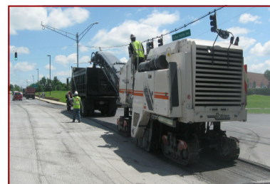
Typical milling operation
