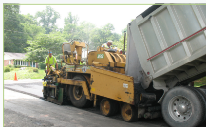
Typical asphalt paving operation
