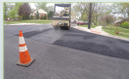
Rollers compact and smooth the asphalt
