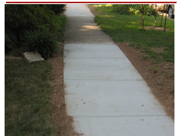
Completed sidewalk repair
